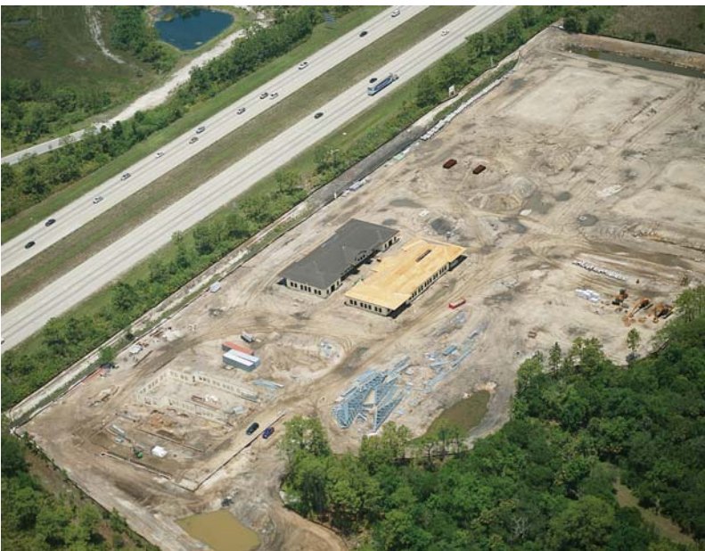
MAY 2006 AERIAL PHOTOS
